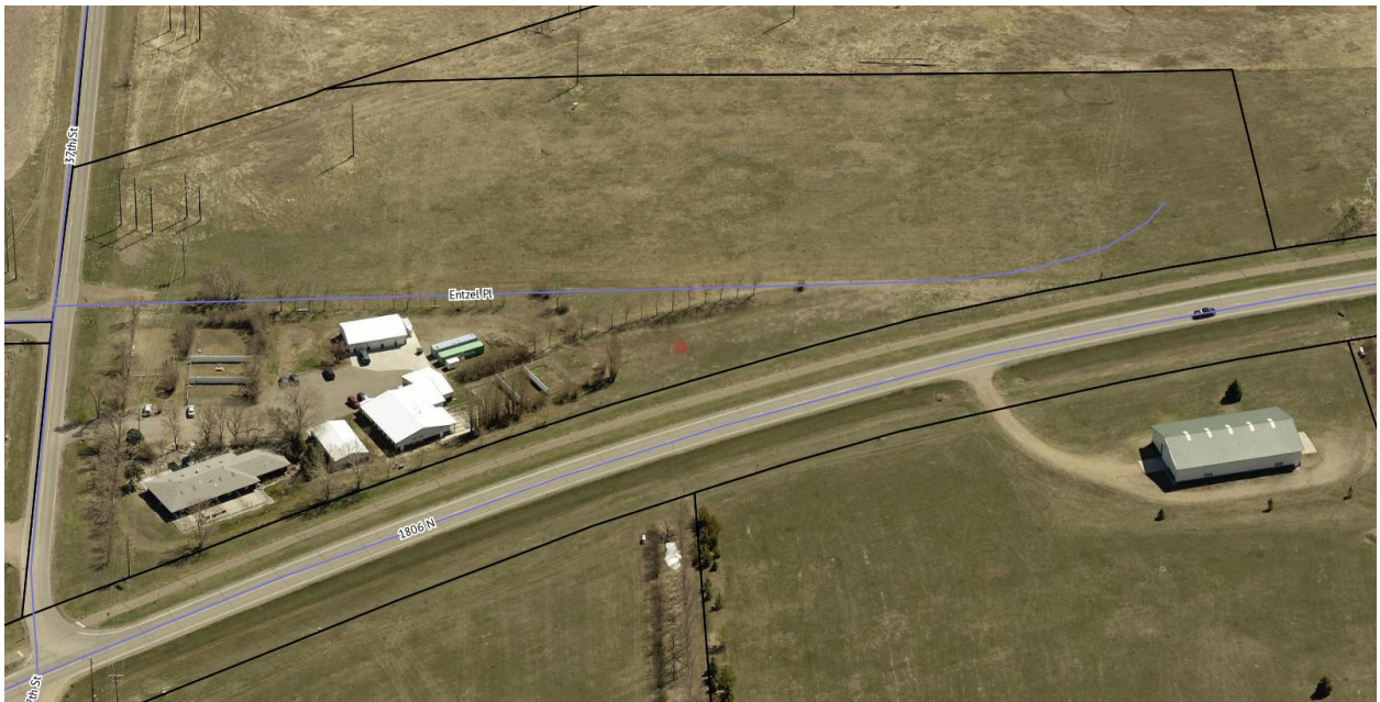
View looking east towards property
