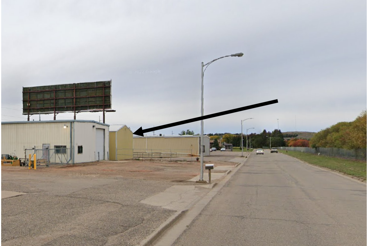
Looking NW down Twin City Drive – arrow pointing at subject building.
