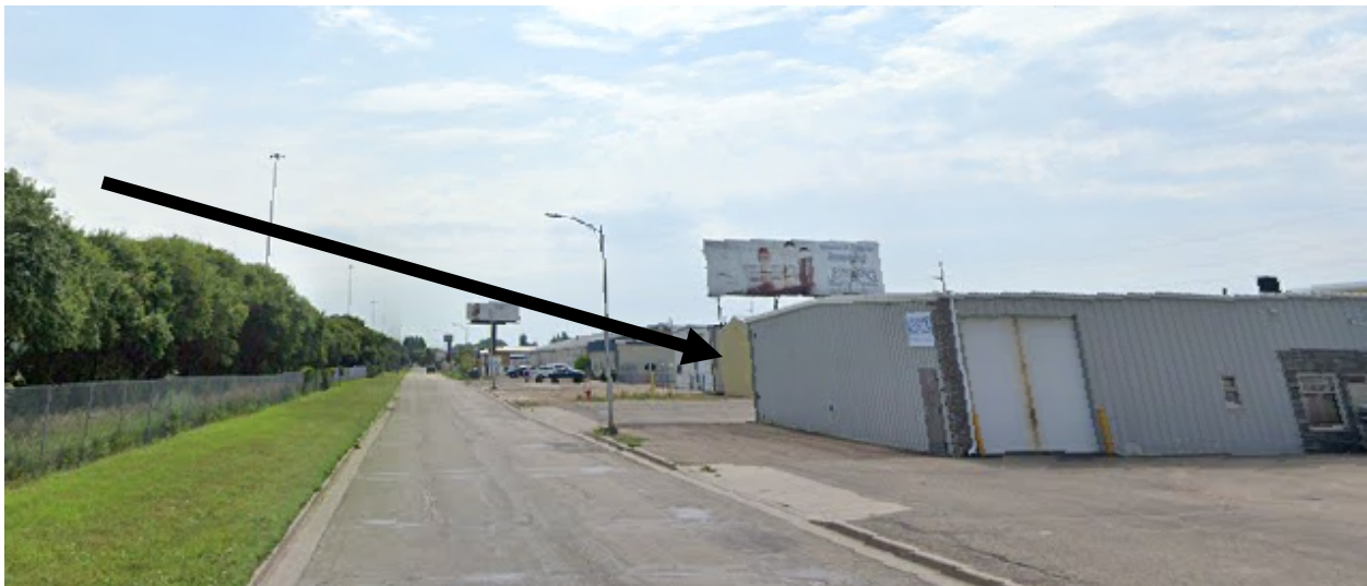
Looking SE down Twin City Drive – arrow pointing at subject building.
