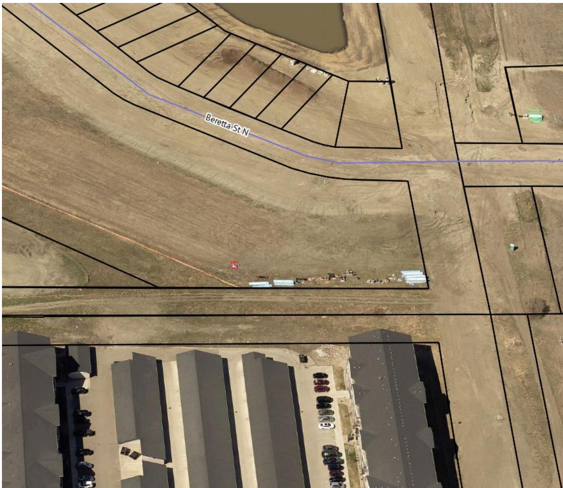
Aerial looking north
