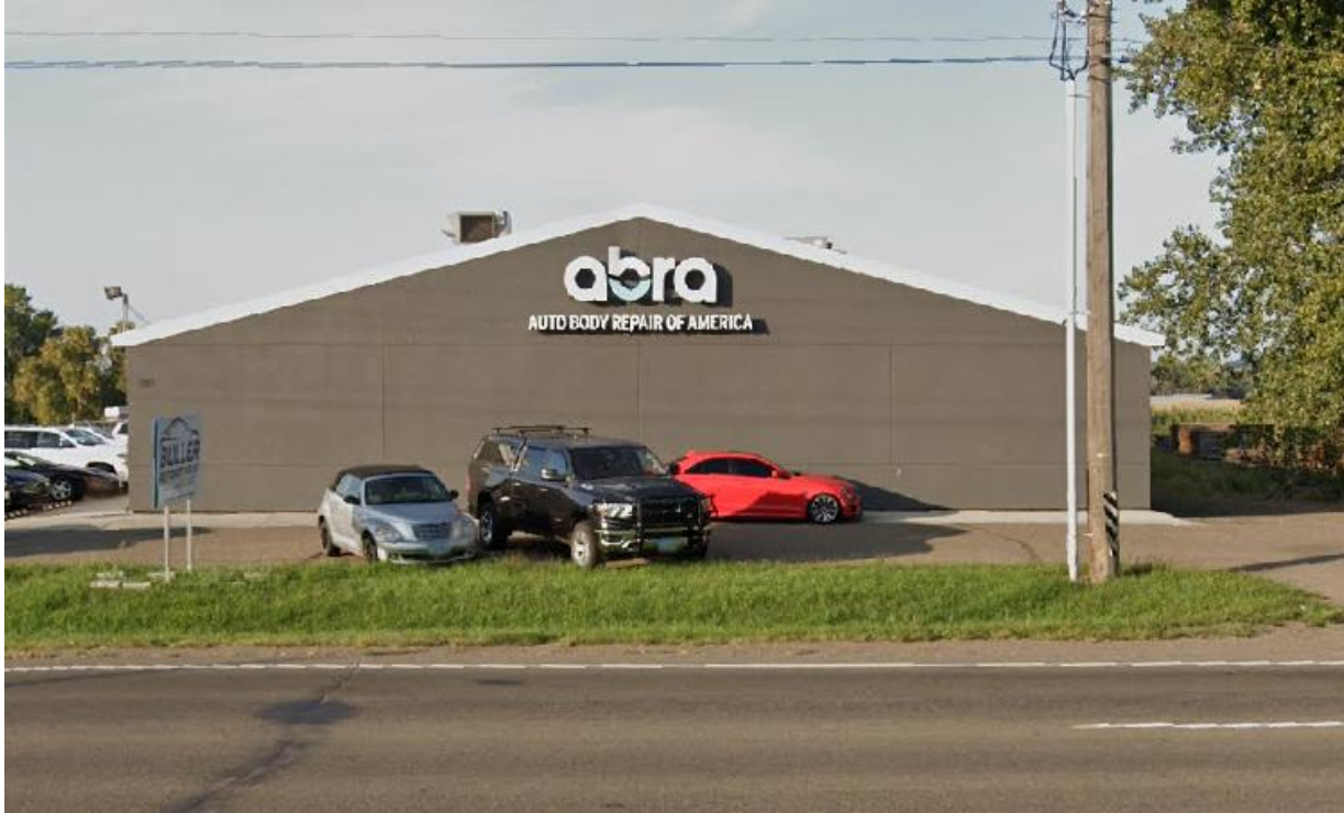
View of existing structure from Memorial Highway SE.
