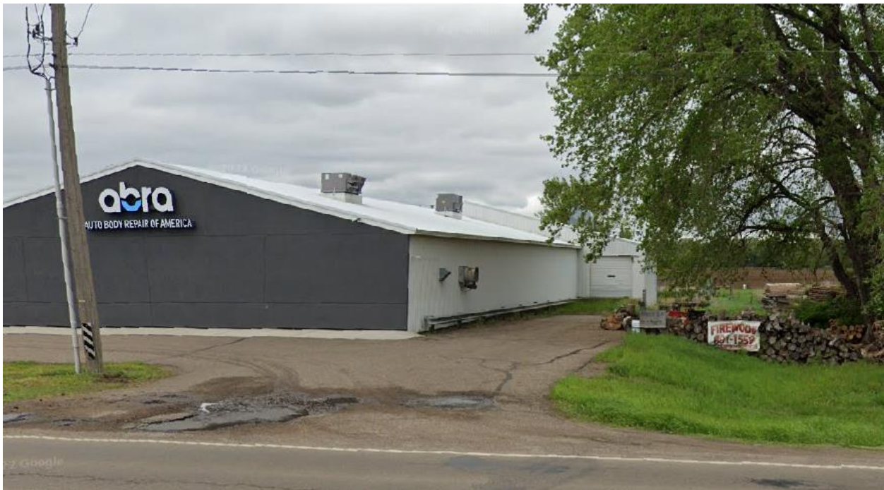
The proposed addition would be built in-line with the loading dock which projects off of the building towards the west (viewer's right).
