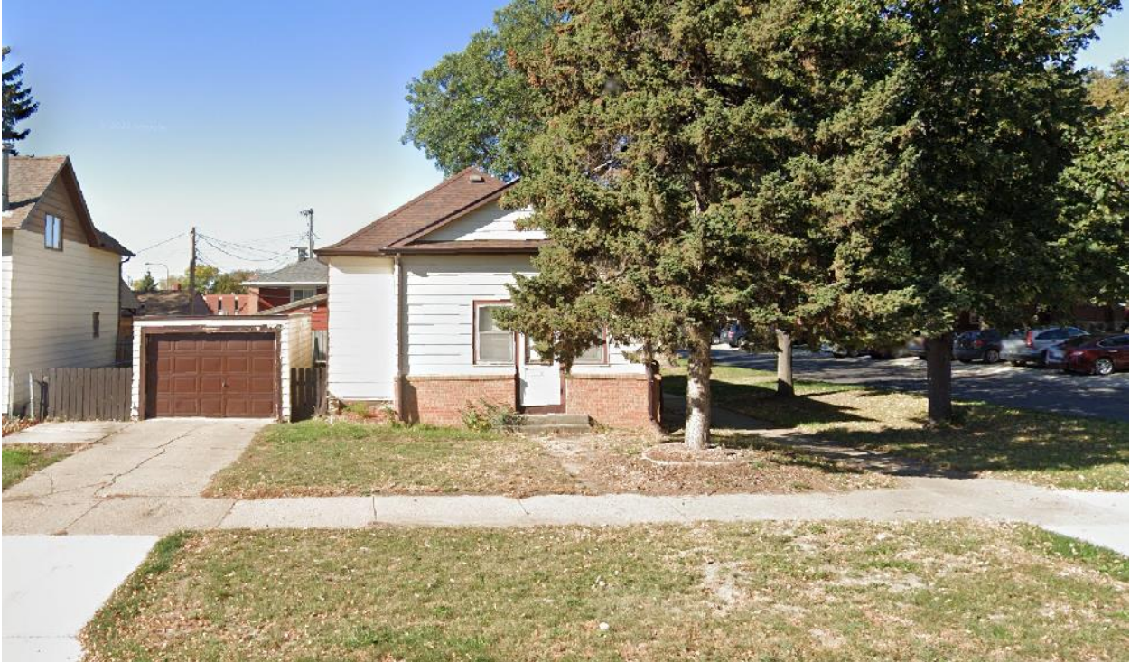
View of existing structure from 1 st Avenue NE
