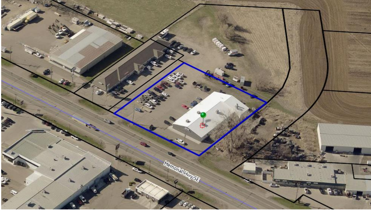
Oblique view, looking south toward subject property. Proposed building addition would be in the rear.
